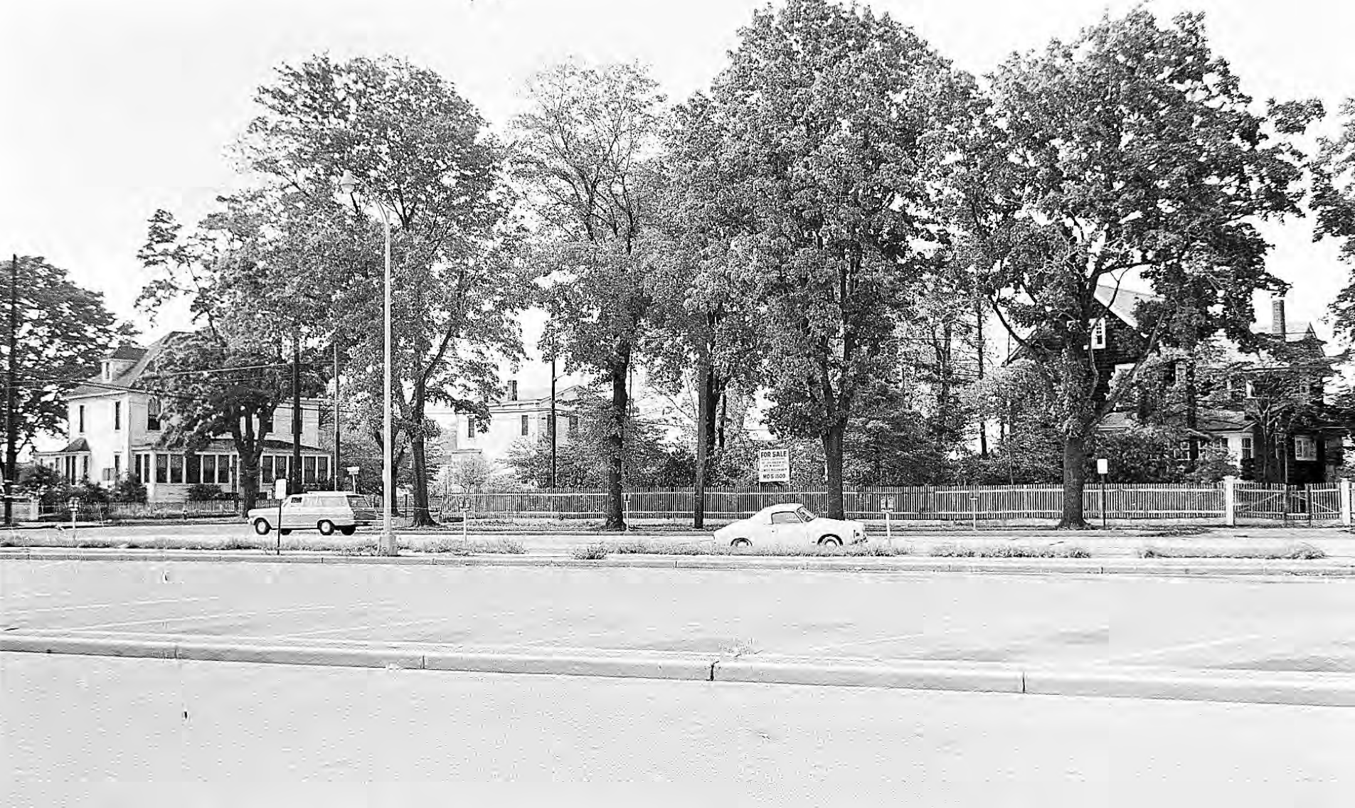
Looking across Marie Street from the Trinity Lutheran parking lot.
