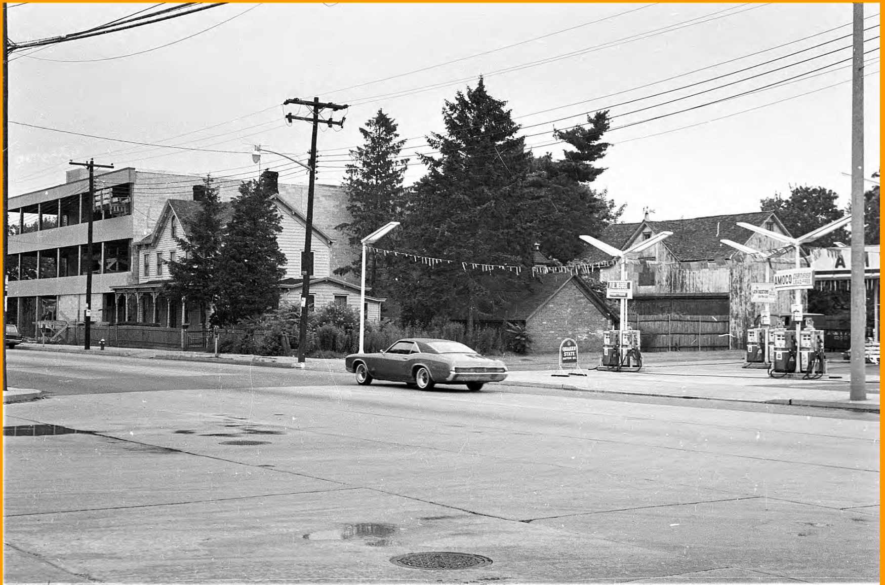
Broadway looking north with Goldman Bros under construction. Old Country Road runs left and right.
