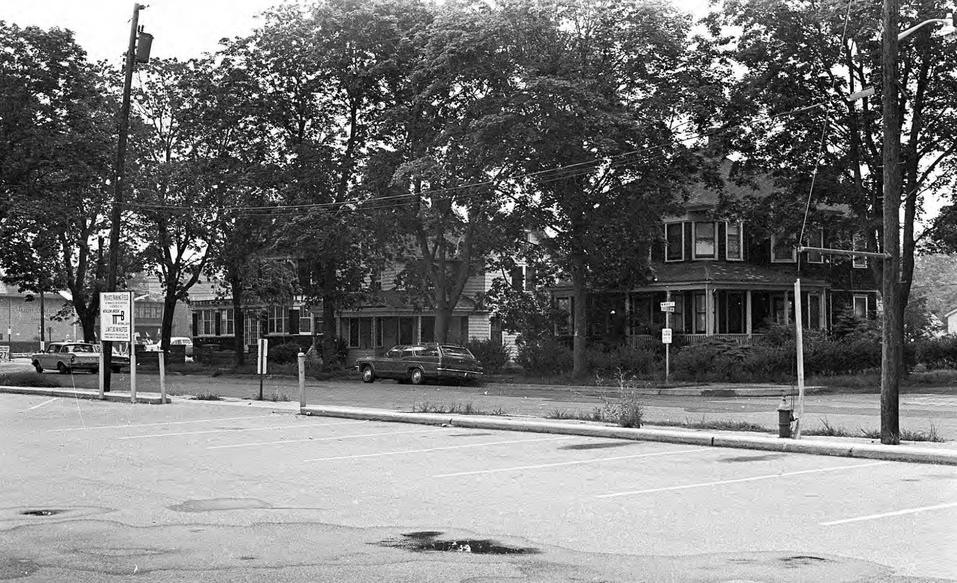
Marie Street looking east toward Jerusalem Avenue. Trinity Lutheran Is visible in the left corner of the photograph.
